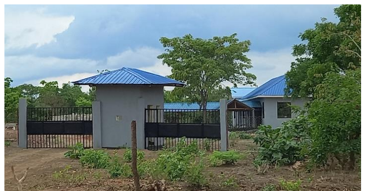
Spiritan Makere health facility still under construction
